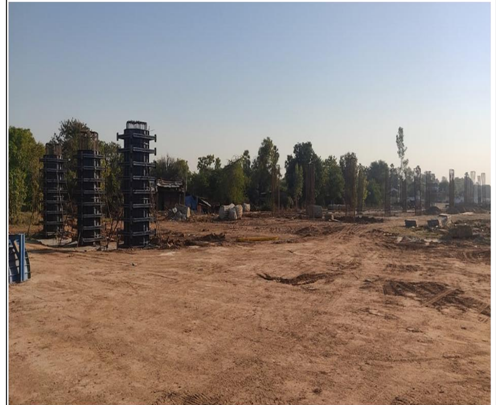
Pier Shaft A1 side LHS MJB @ 352+281
