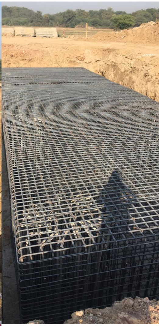
Pile Cap reinforcement binding work of Major Bridge
