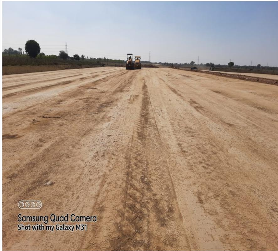
SG top layer rolling in progress at ch 360+600 to 360+720 LHS
