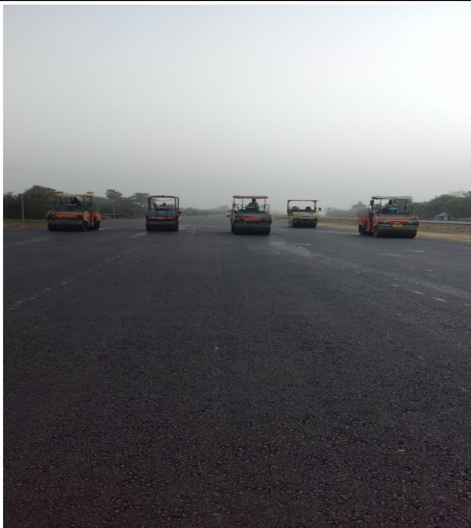
Laying of DBM-1st from Ch. 353+450 to 354+020-RHS
