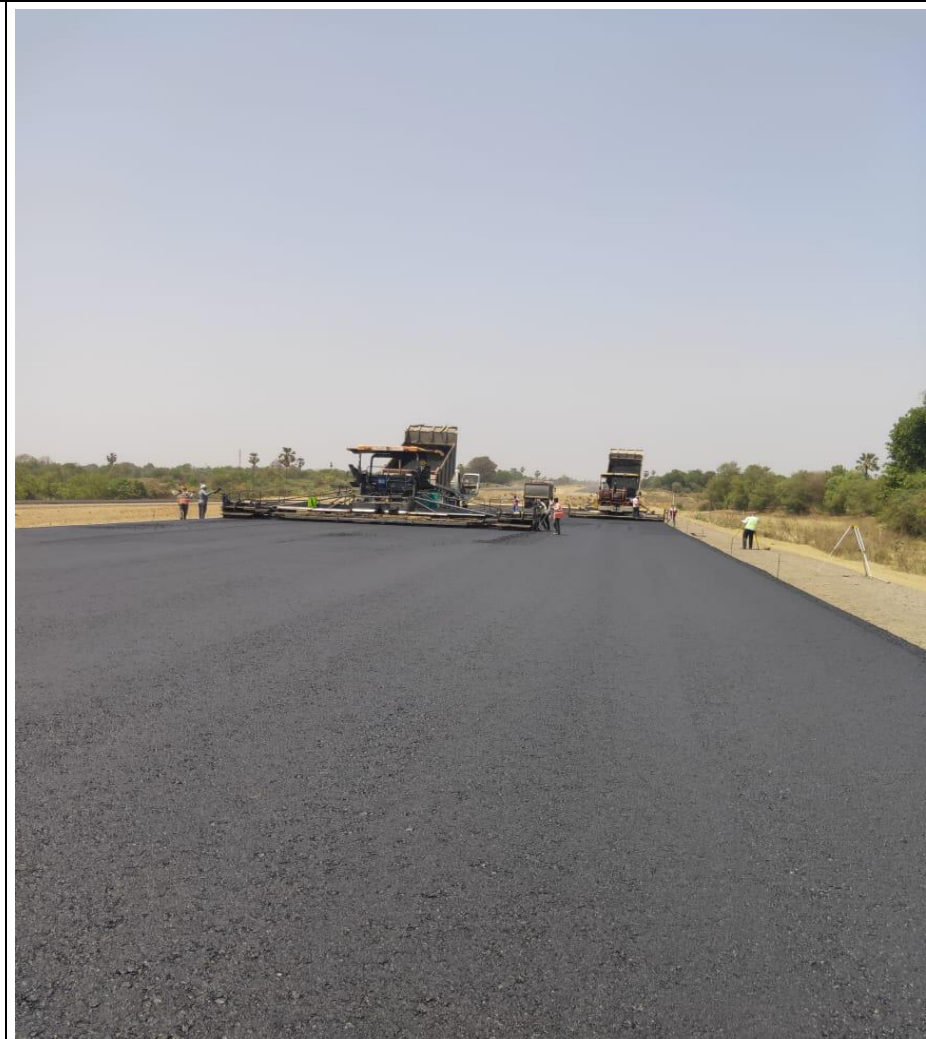
Laying of DBM-1st from Ch. 358+170 to 358+450
