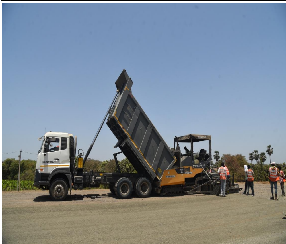
WMM laying from ch. 356+060 to 356+400 RHS
