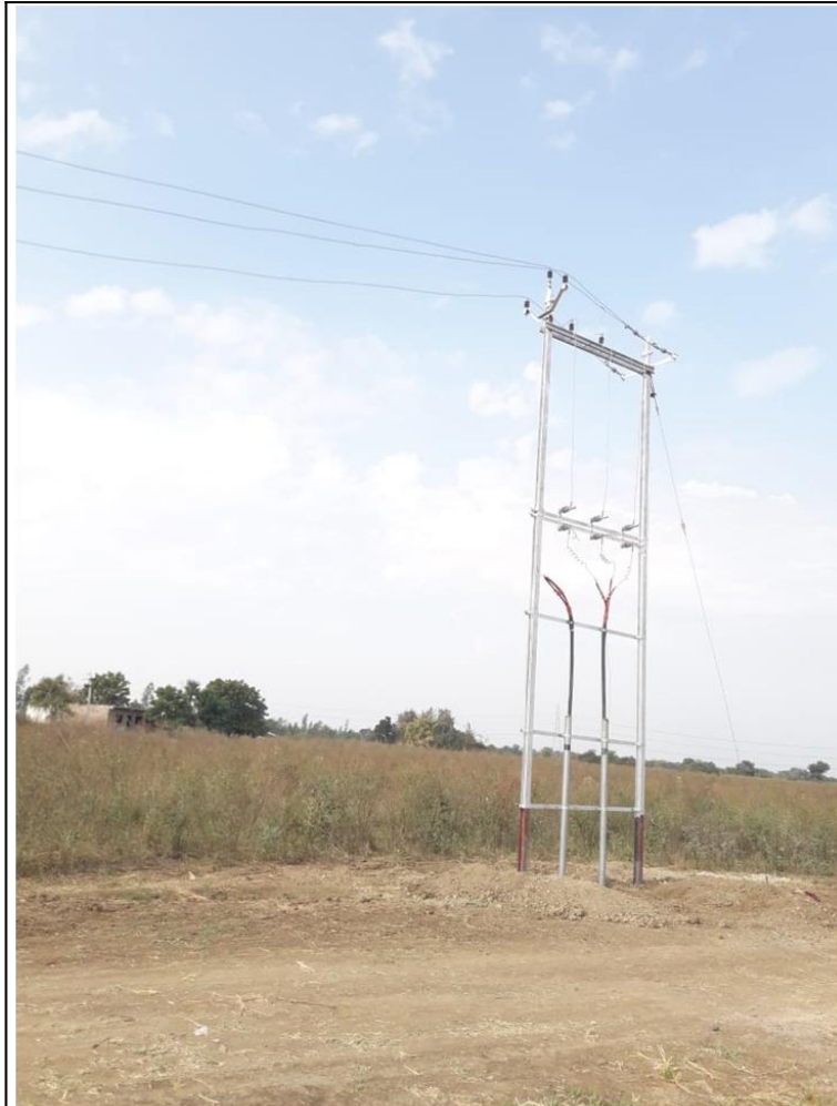
Utility Shifting- Electric line charging at ch.362+650
