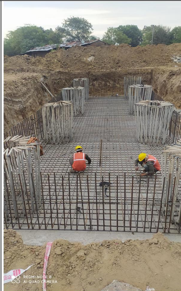
Pile Cap reinforcement binding at MJB 352+281
