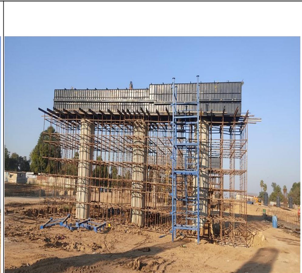
Pier Cap –P-5 RHS A-1 side MJB @ 352+281
