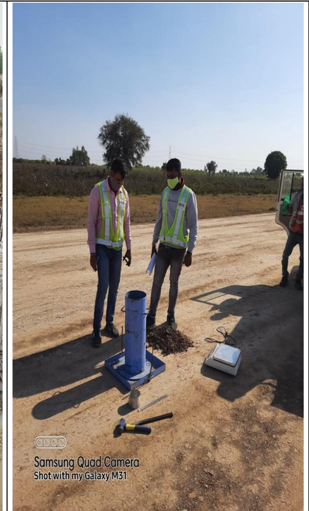
SG top fdd at ch.-360+ 600 to 360+ 720 LHS
