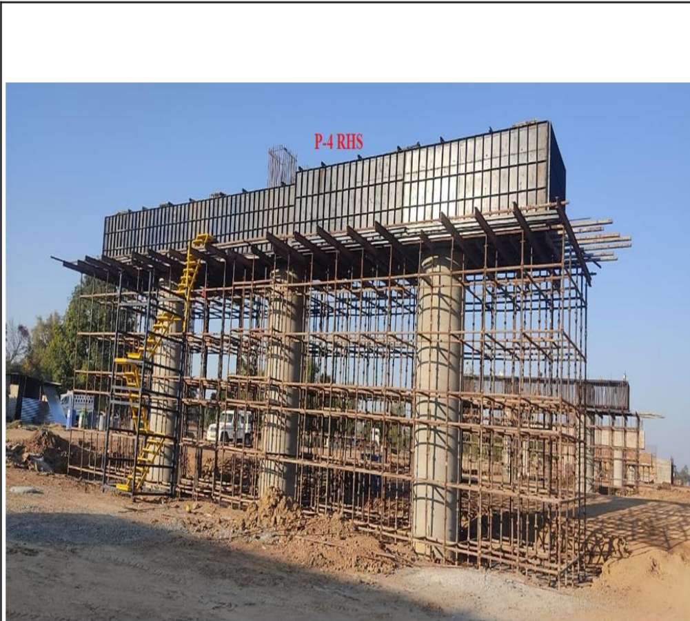
Pier Cap –P-4 RHS A-1 side MJB @ 352+281
