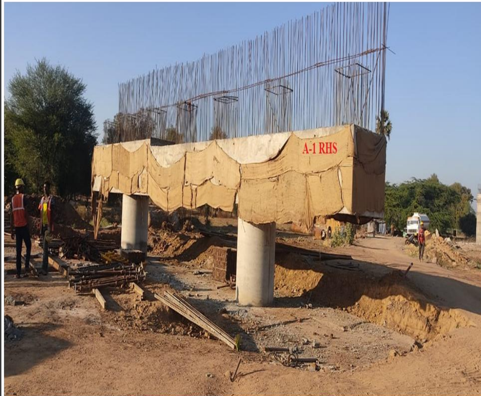
Abutment Cap –A-1 RHS A-1 side MJB @ 352+281
