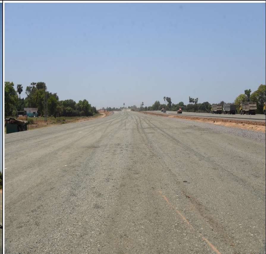
WMM laying from ch. 356+060 to 356+400 LHS
