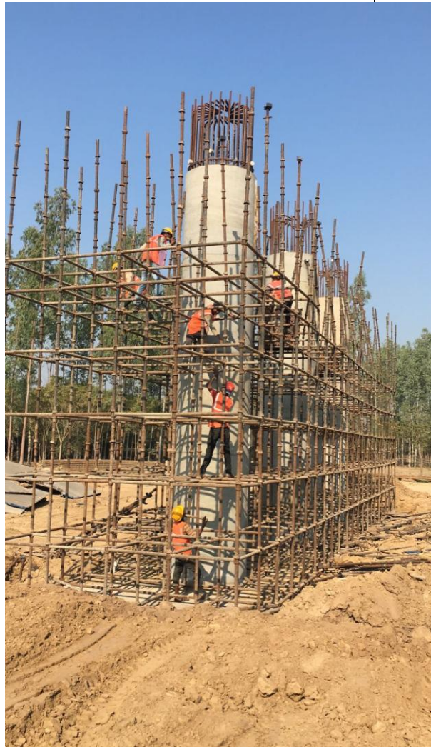
Staging & Shuttering Work for Pier Cap & Pier Shaft
